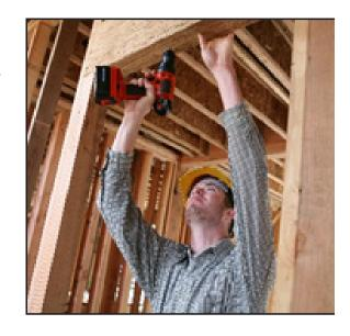
Electrically powered tools present additional risks. Shocks and burns from an improperly grounded tool, or making contact with exposed wiring, may result in electrocution or severe injuries. Workers can be seriously injured or killed from shocks that cause them to fall from ladders and elevated work surfaces.
