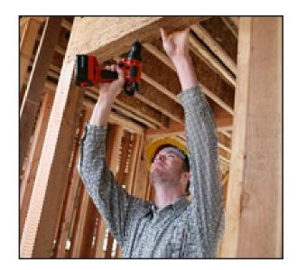
Electrically powered tools present additional risks. Shocks and burns from an improperly grounded tool, or making contact with exposed wiring, may result in electrocution or severe injuries. Workers can be seriously injured or killed from shocks that cause them to fall from ladders and elevated work surfaces.
